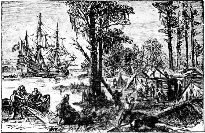
BUILDING TENTS AND BOOTHS AT JAMESTOWN
